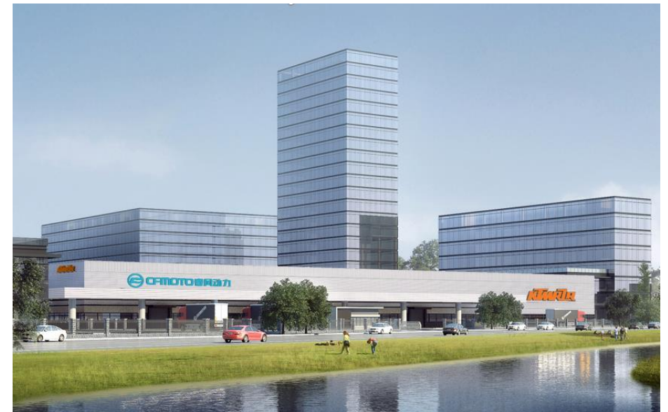
Plant under construction
